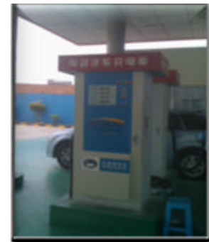
Fig B2: 180 kW Fast Charger at BYD in Shenzhen
